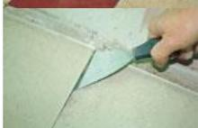
It is necessary to remove or to fix back all the parts that sound hollow (tiles etc).
