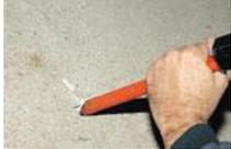
In case of old screeds (friable, low quality etc) probe hardness through its entire thickness. The screed must be cohesive.
