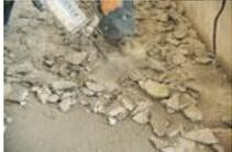
If the top layer of the surface is not hard enough, you have to remove it to obtain a sound surface.
