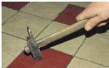
**Glued or sealed coatings.** Check the adherence of old tiles and slabs with a hammer or a spatula.
